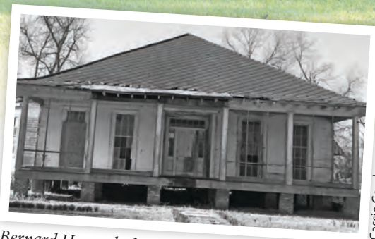
Bernard House, before renovation
