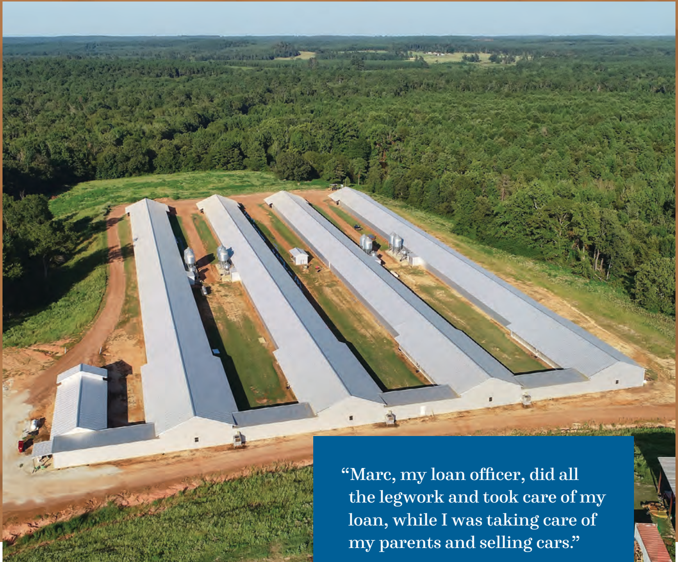
Four new 600-foot-long poultry houses, financed by Legacy Ag Credit, shine in the evening sun at Witcher's Flat Creek Farms in northeast Texas.
